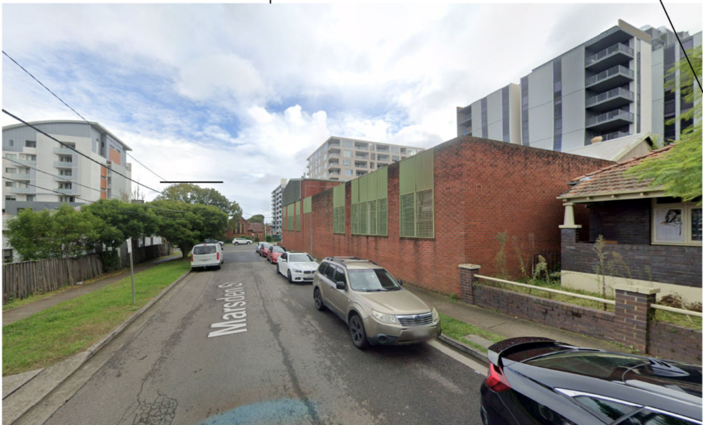
VIEW TO SITE FROM MARSDEN ST
